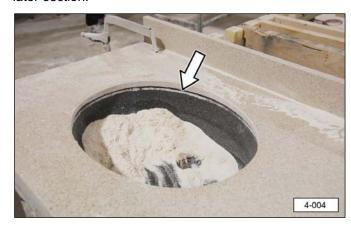
4. Inspect the seam between the sink and countertop, looking for any voids or cracks. If defects are found, the sink should be removed and reglued.
