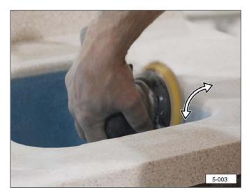
2. Use 220 grit sandpaper to remove sanding scratches and open up the surface to fully reveal the Swanstone pattern. Sand the entire surface of the sink and countertop.
