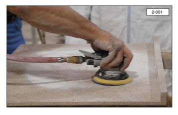
6. Thoroughly sand the rim of the sink with 36 grit sanding pads. Remove all gloss and rough up the surface to allow for proper adhesion.
