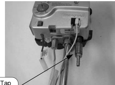
Pressure Tap Shown Installed
