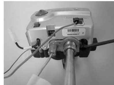
Gas Control shown in the "OFF" position
