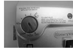
Gas Control shown in the "OFF" position
