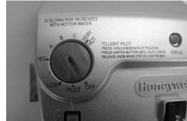
Rotate knob counter-clockwise to the “OFF” position.
