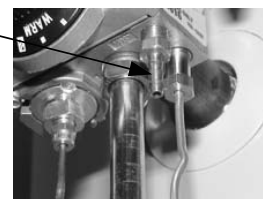
Pressure Tap Shown Installed
