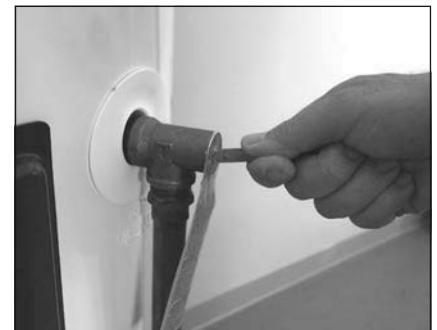
Figure 46 - T&P Relief Valve
