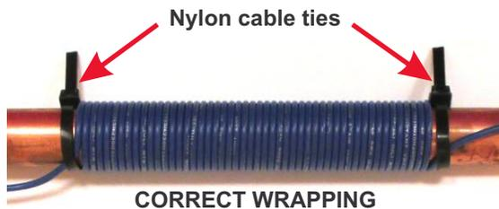
Make sure the wraps are flush against one another, wrapped tightly and not overlapping, except for the second layer that is required on all copper pipe.
