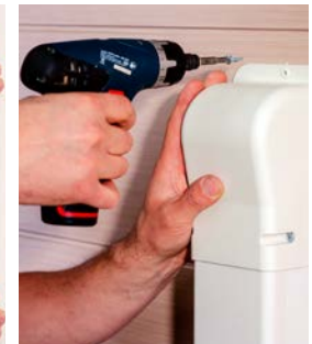
5. Install the top fitting using the included stainless steel screws for a rigid assembly.
