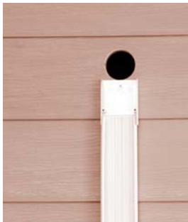
1. Affix the bottom half of the fitting and duct to the wall (screws not included).
