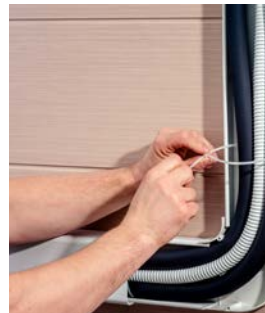
3. Place the line set, drain hose, and control cable within the duct. Fasten the cable tie.
