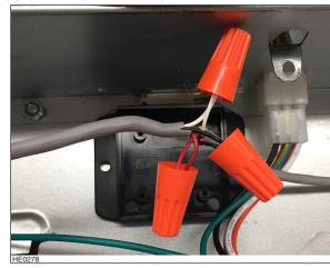
Put the wire nuts inside the connection box base, then snap the connection box lid on its base, ensuring the ADA cable runs through the open notches.
