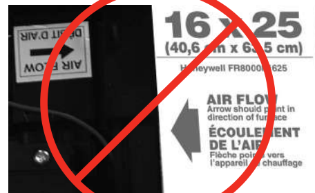
Fig. 18: Make sure that the arrows on the filter point in the same direction as the arrow on the enhancement module. This will be in the same direction as airflow.
